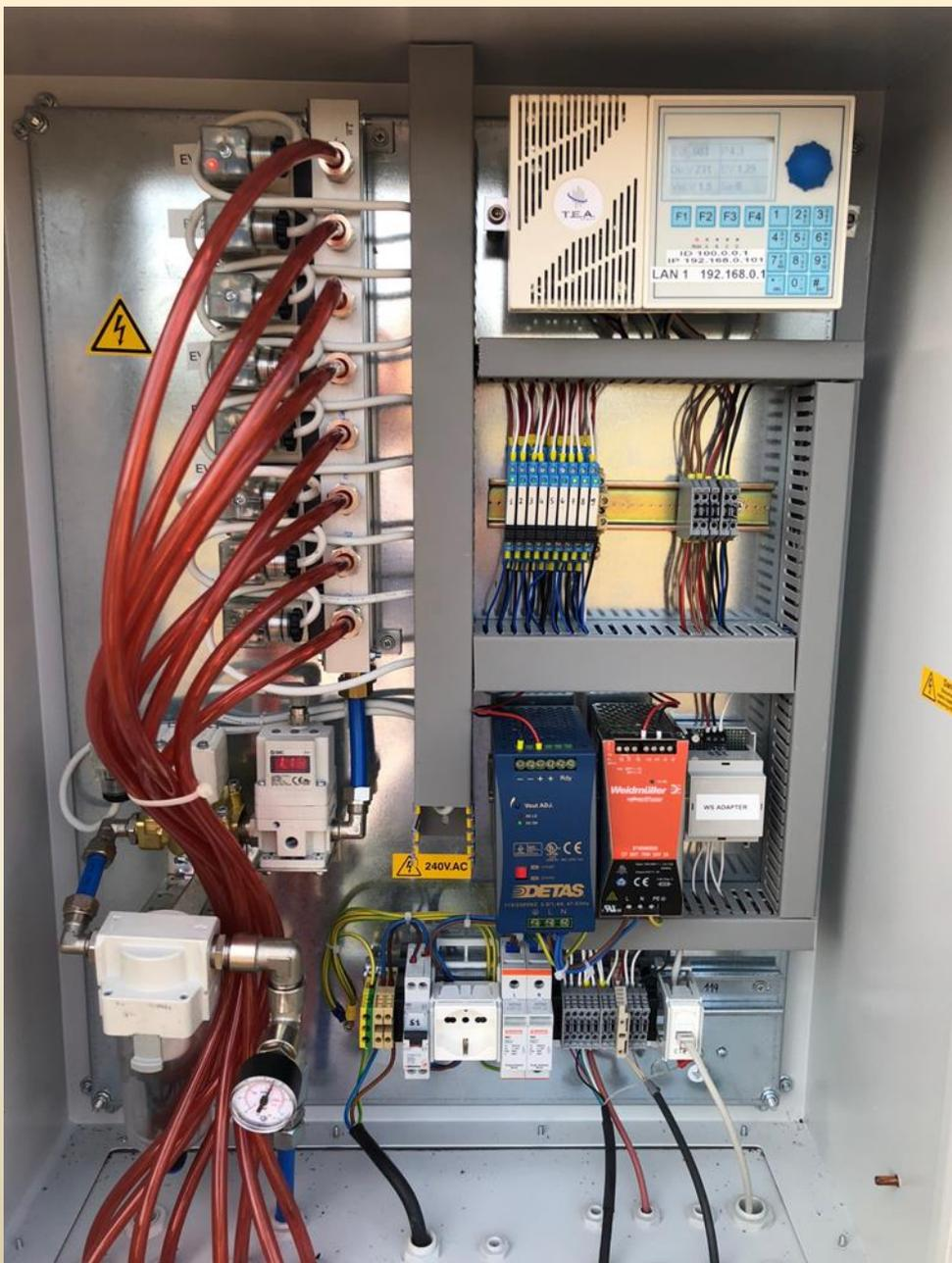
The heart of the control unit is a CPU that control and display the ring functionality and its regulation.
