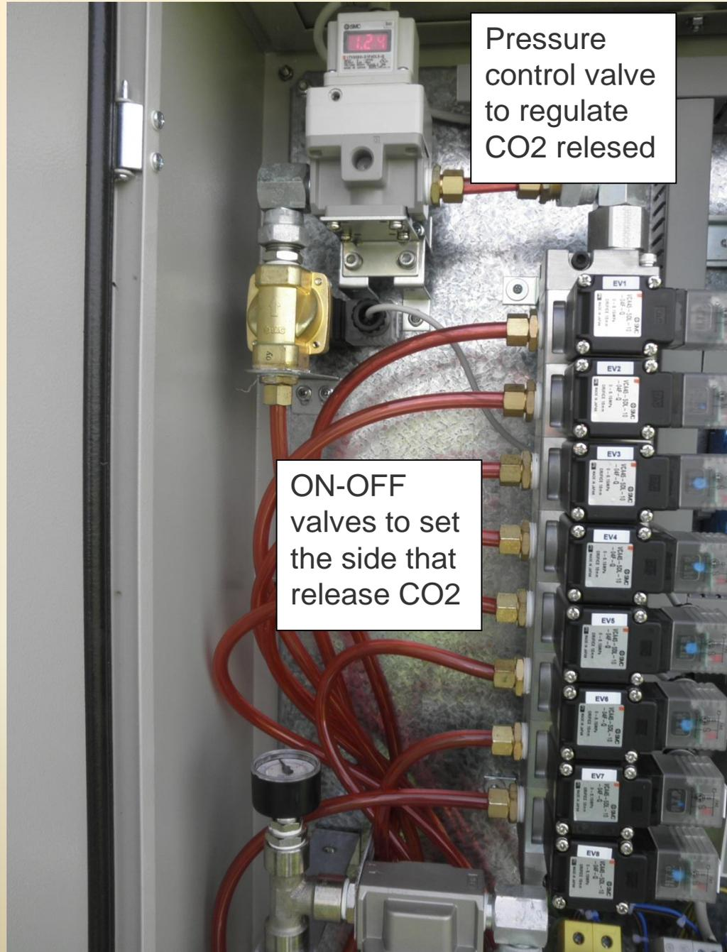
Pressure control valve to regulate CO2 released
